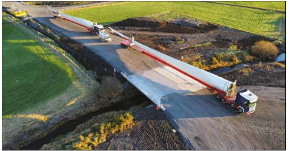
Turbine deliveries underway to the Yellow River site.
