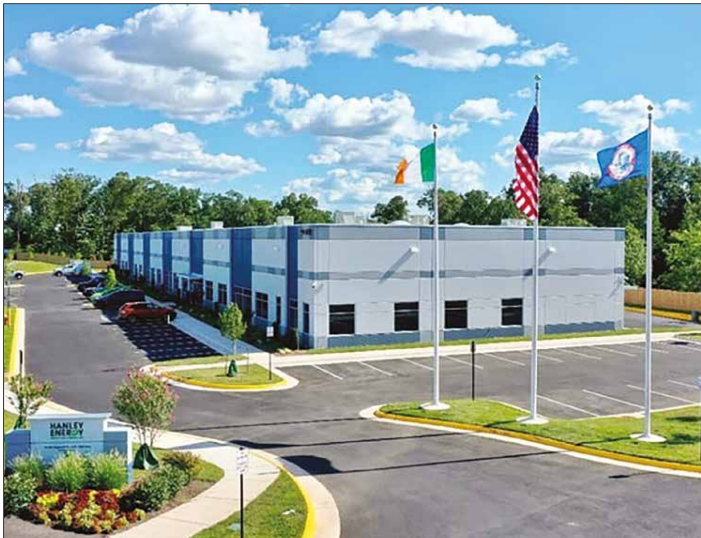
Hanley Energy has invested $12m in its new facility in Virginia, USA.
