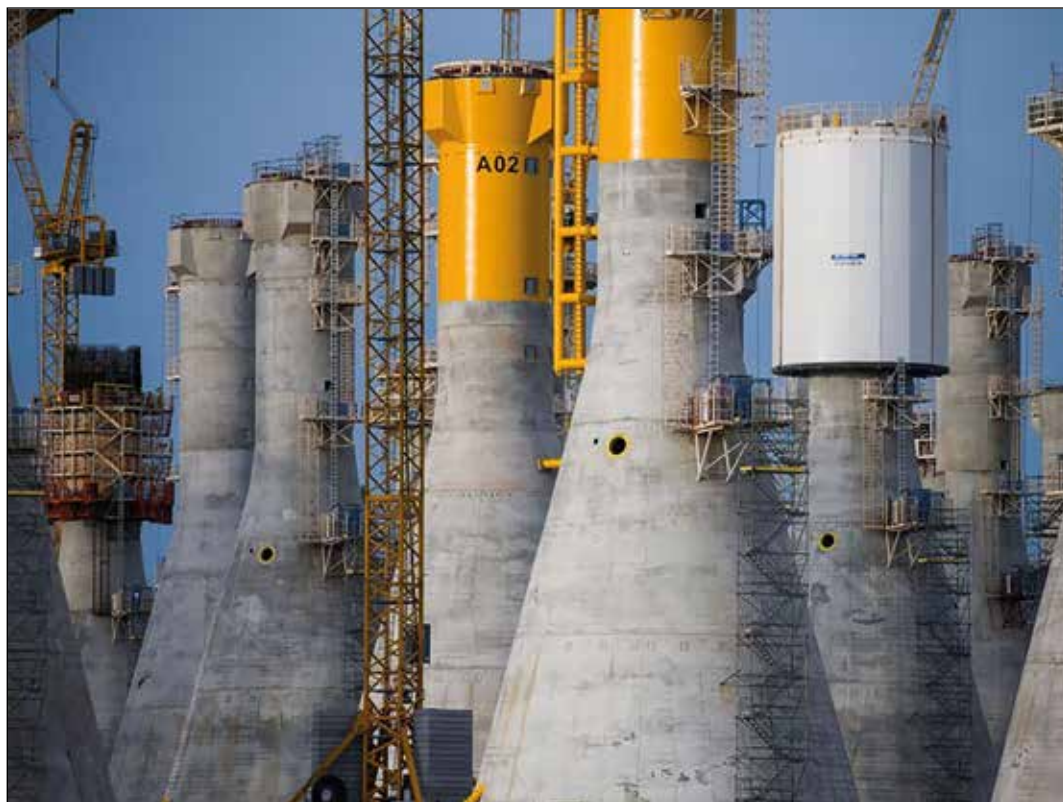
We have the energy solutions for green power, but we need commitment and public support. Cranes seen at the construction site of gravity-based wind turbine foundations for the Fecamp offshore wind farm.
